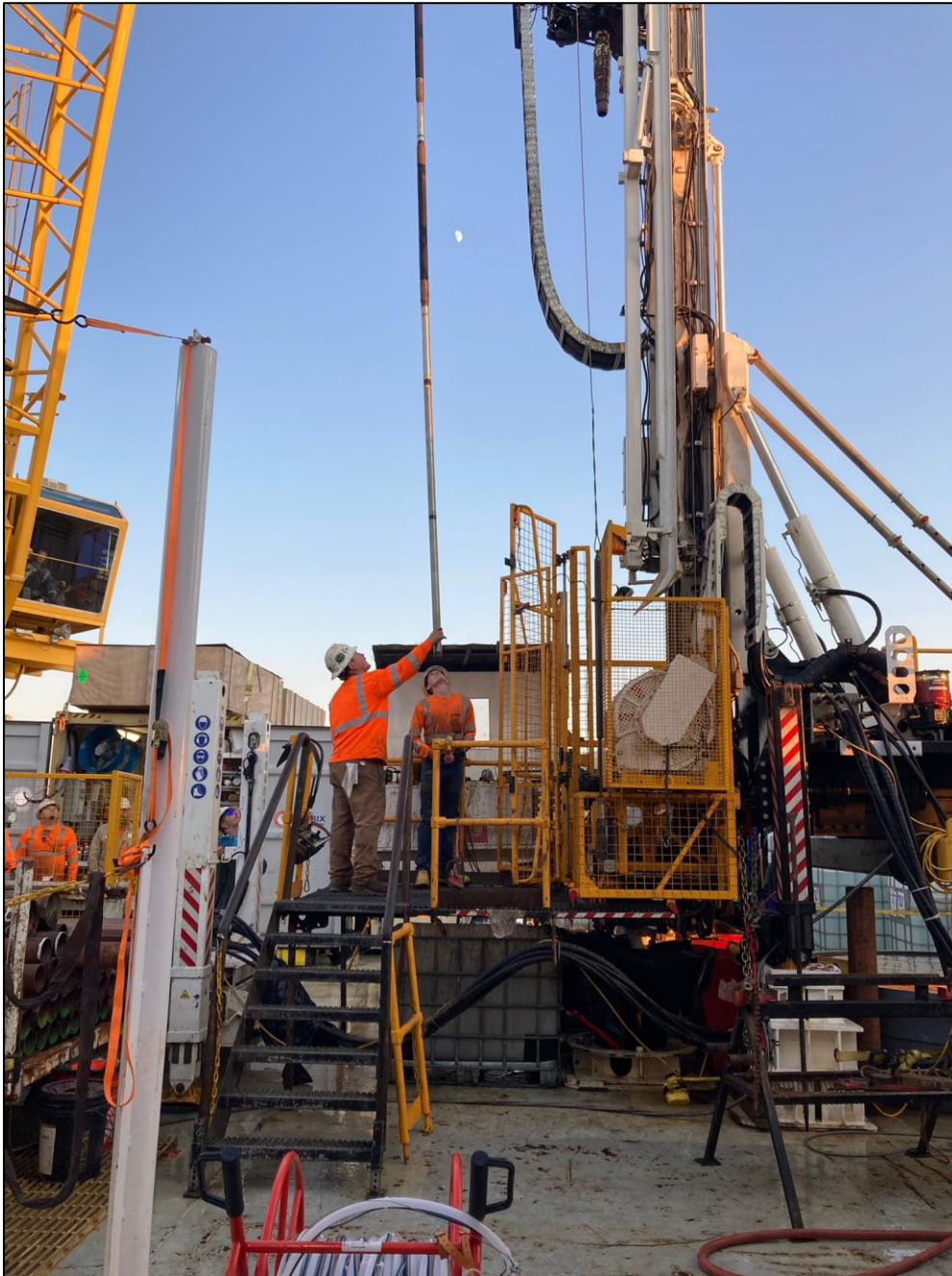
Figure 1 Installing the packer in the borehole. The packer isolates the sediments containing the groundwater we want to pump. ROBINSON@ECORD_IODP3_NSF_packer.
