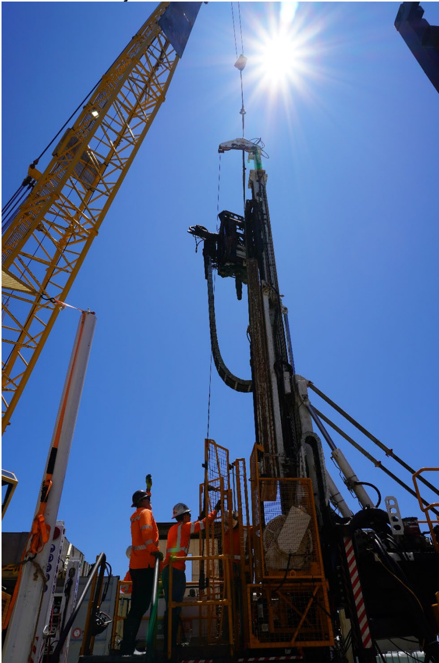
Figure 1: The drilling team deploy the packer downhole in preparation for the pump test at Site M0113A (photo Brickell@ECORD_IODP3_NSF_Packer_install_24.07).
