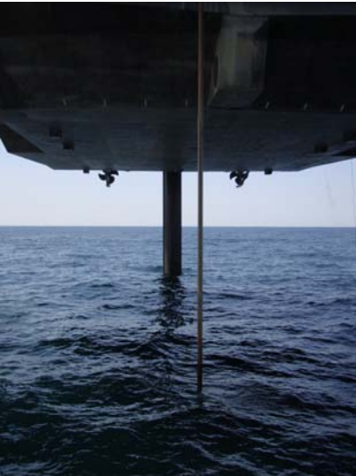
Under the L/B Kayd , looking from the bow to the rear leg. The thin pipe in the foreground is the drill string lowered from the drill rig.
