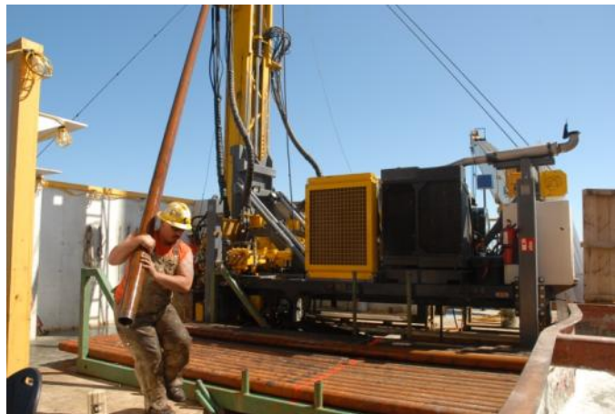
Jay brings the pipe back down into the pipe rack after tripping it out (J-N. Proust©ECORD/IODP).
