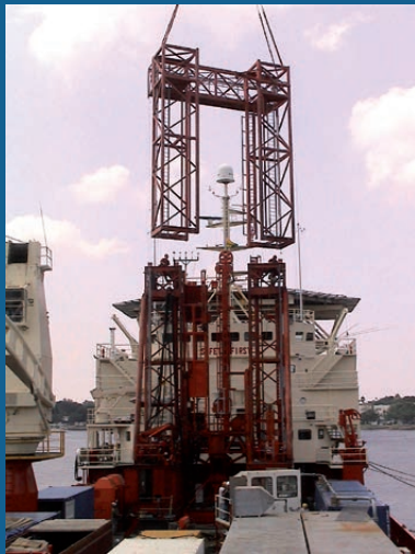
Assembling the derrick onboard the DP Hunter - Exp 310 Tahiti Sea Level .
